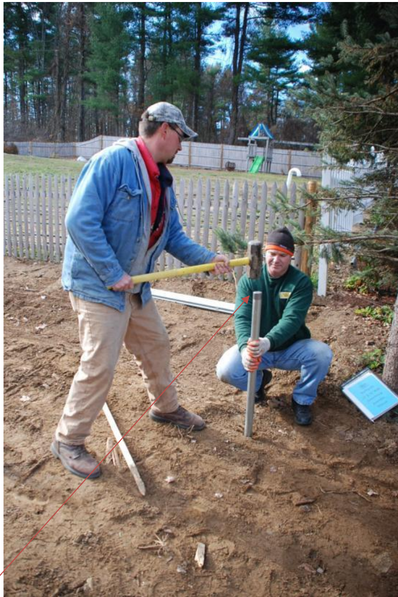
This is the ground post driver inserted into the ground post
